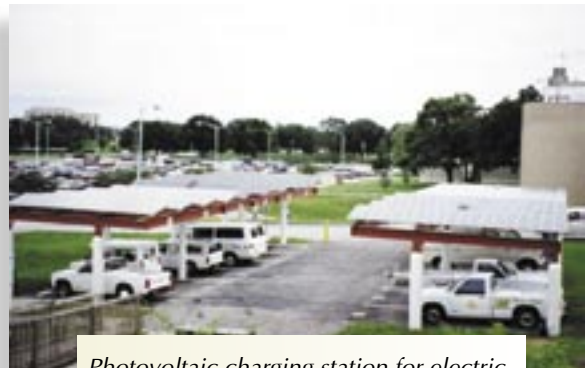
Photovoltaic charging station for electric vehicles at University of South Florida.
